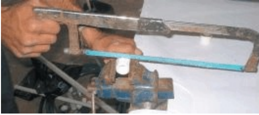
Cut the thread off the female adapter
