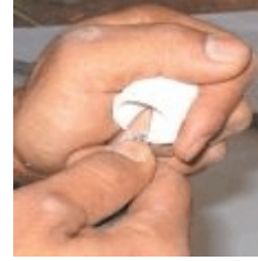
Clean the non-threaded part with a knife
